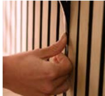
With the white strip on the LED light facing the felt, start pushing your first light strip into the slat gap, starting from the bottom edge of your panel.
