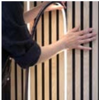
If your panel has a wood veneer, we advise against rubbing your hand along the surface, to avoid splinters. Simply press a small section in at a time with your palm or thumb.
