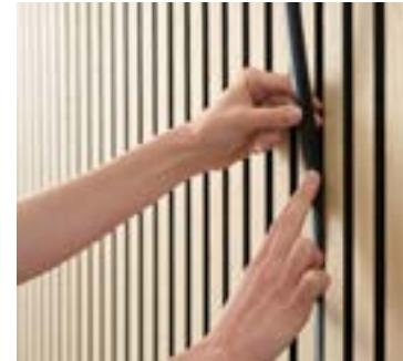
Use your hand to firmly press the strip snugly between the slats until the surface of the lights are exactly flush with the surface of the slats.
